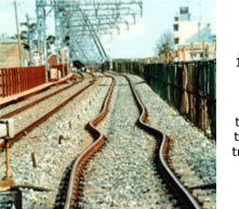
This photograph was taken after a 1995 earthquake in Japan. A seismic wave transferred enough energy through the ground to bend the railroad tracks, leaving them in the shape of a wave.
